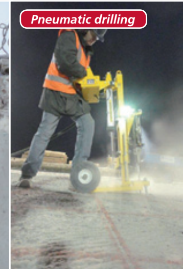
Coentunnel, cracking of 2,000 piles
