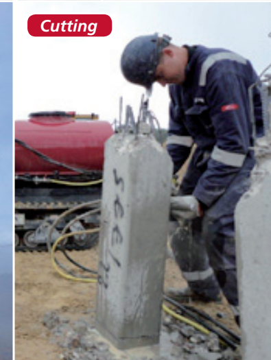
Pneumatic drilling of holes
